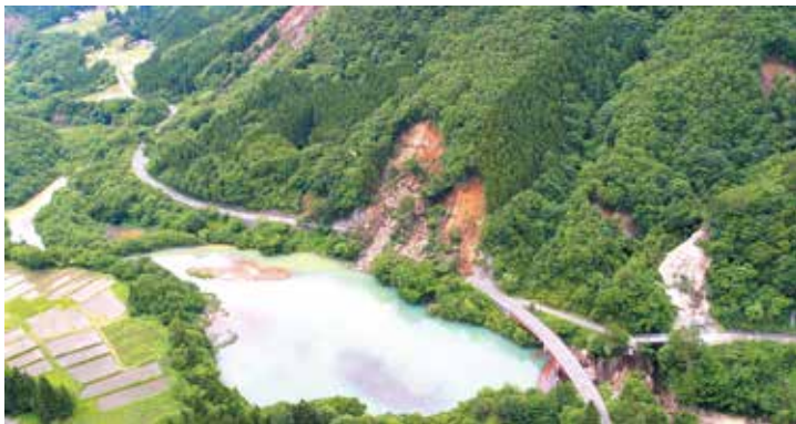
▲ Landslides: The Iwate-Miyagi Nairiku Earthquake, 2008 *Photo provided by Iwate Pref.
