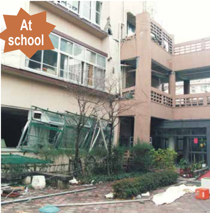
▲ School buildings damaged by an earthquake: The Great Hanshin-Awaji Earthquake Disaster, 1995 *Photo provided by Kobe City
