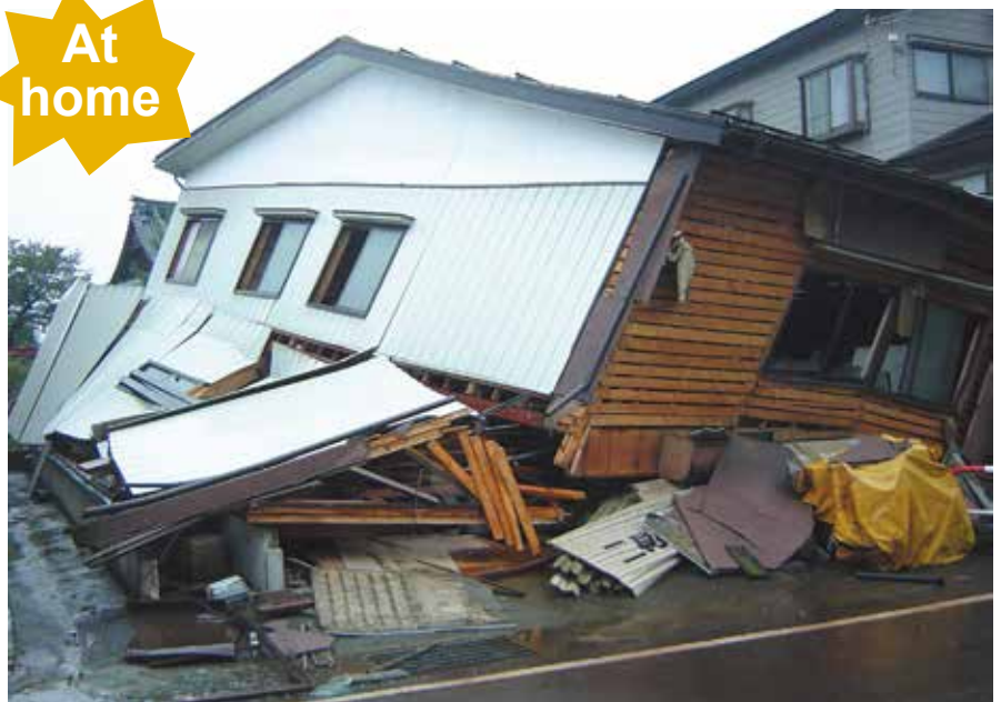
▲ A house whose ground floor was crushed completely: Niigata Chuetsu Earthquake, 2004 *Photo provided by Tokyo Metropolitan University
