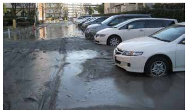
▲ Liquefaction: The Great East Japan Earthquake Disaster, 2011 *Photo provided by a voluntary disaster prevention troop from the Tomioka Estate Housing Management Association of Urayasu City, Chiba Pref.
