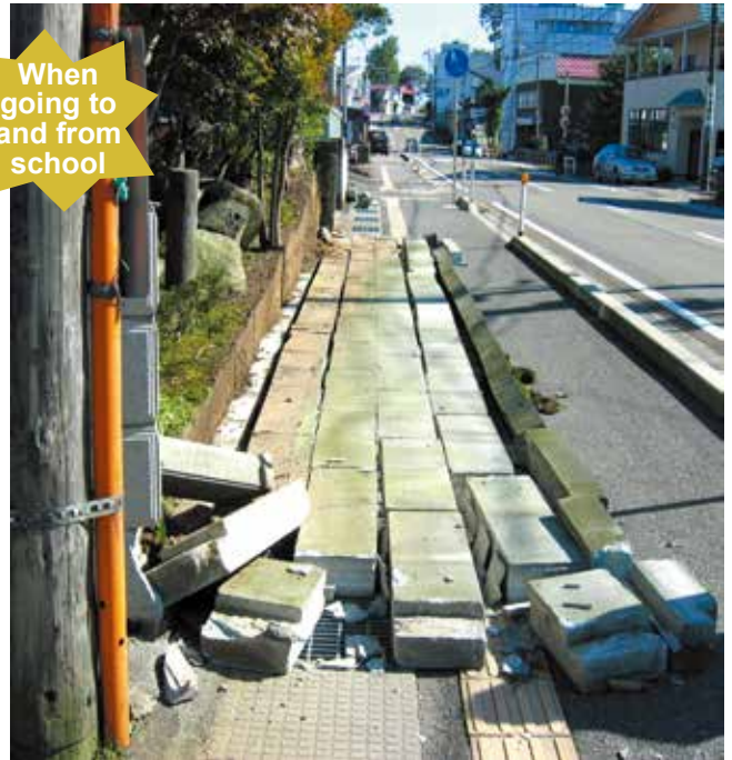
▲ A concrete block wall collapsed by an earthquake: Niigata Chuetsu Earthquake, 2004 *Photo provided by Tohoku University
